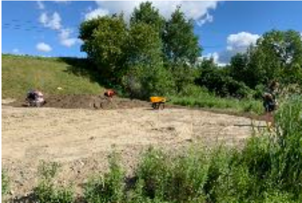
Getting ready for sod
